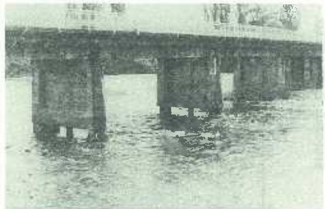
Fig. 4: Wairoa bridge at Brightwater.
