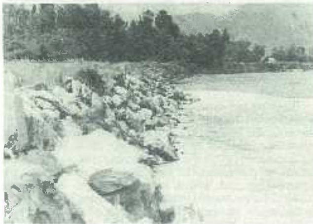
Fig. 1: Rock protection on eroding banks of the Wairoa and Waimea rivers.
