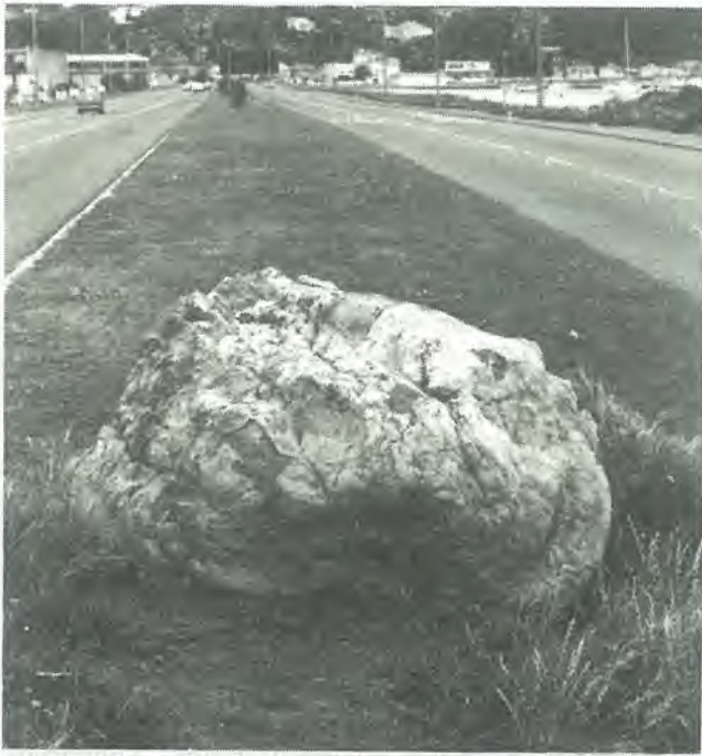
Fig. 5: This rock has been struck on two occasions, causing five people to be seriously injured. Note how the rock was shifted by the last impact.
