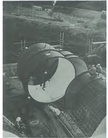
Penstock at Maraetai II during erection, showing a vinyl interior.
