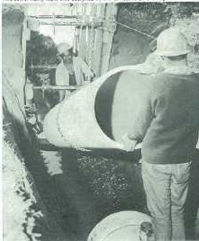
Pipe is lowered into trench ready for jointing.
