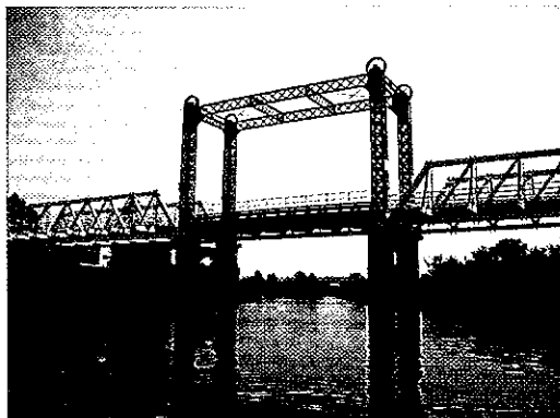
The Hinton Bridge crossing the Paterson River Hunter Valley, NSW
