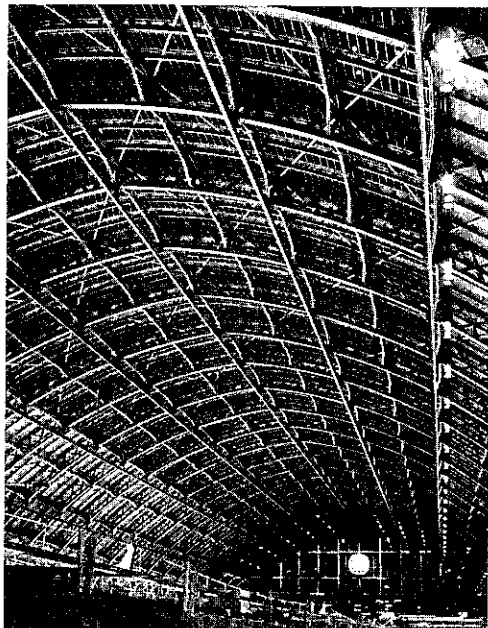
St Pancras Roof (March 2007 – the refurbished St Pancras station roof) © R J M Carr
